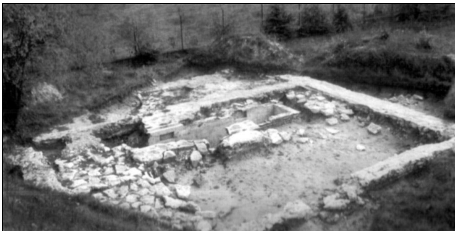
Document 13: Photograph of the remains of building D. 10
