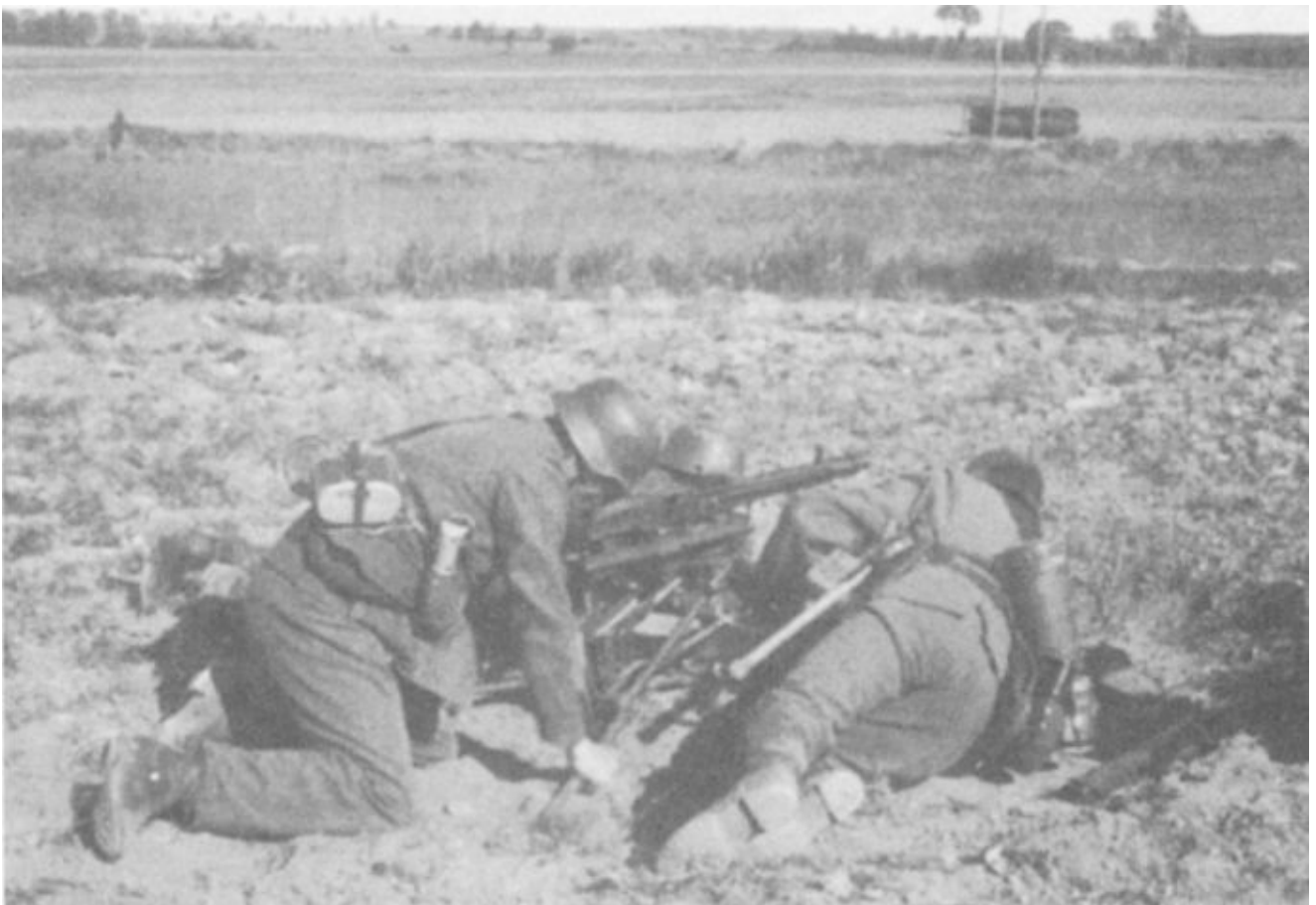
A machine-gun team in position.
