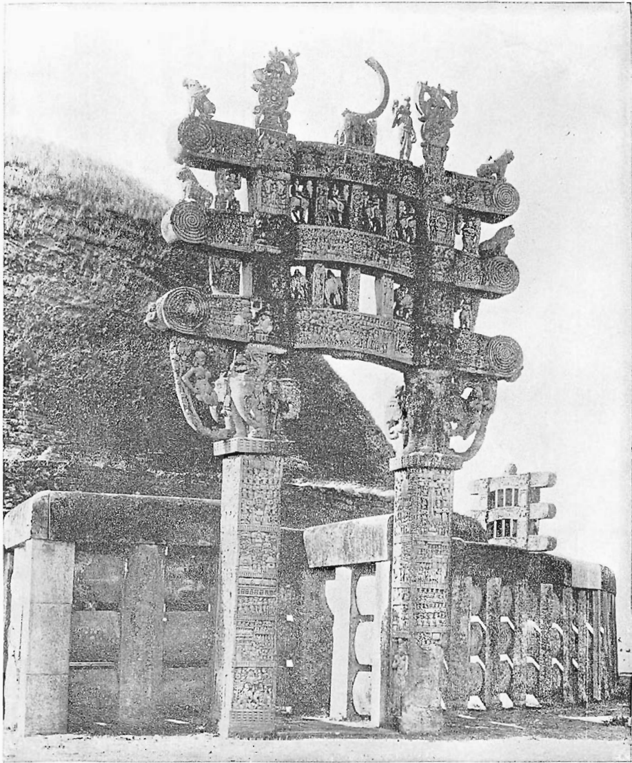
FIG. 51— Sanchi Stupa, north gate Underwood & Underwood
