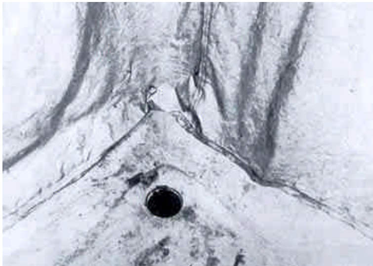
Drain in the corner of execution cell.
