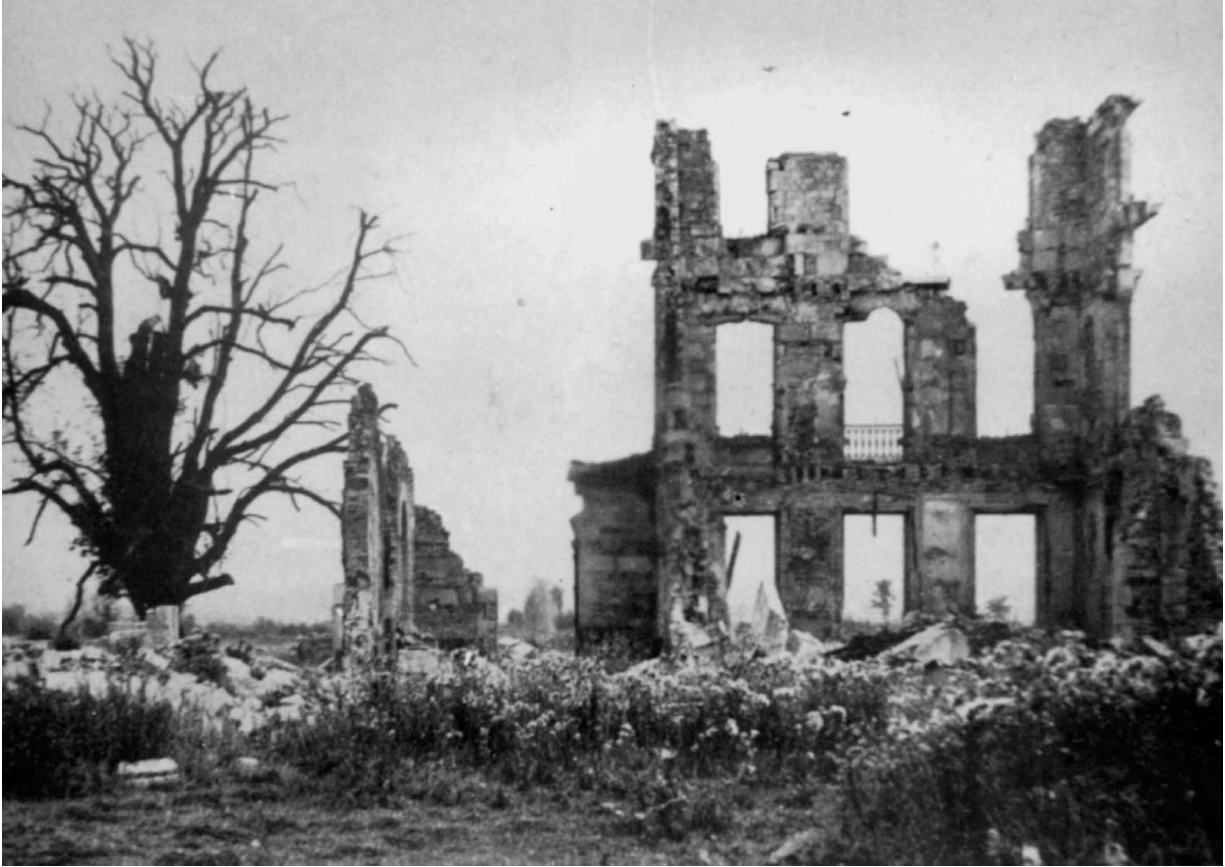
The ruins of Château Boislonde testify to the severity of the fighting.
