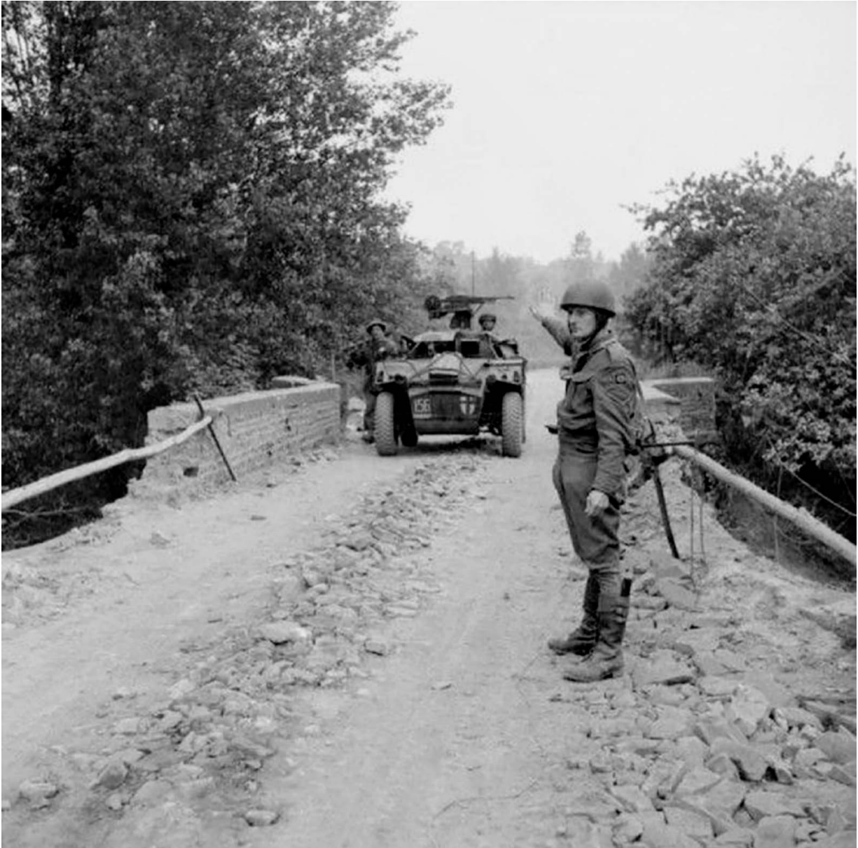
The narrow Tourmauville bridge damaged by tanks in the hands of a military policeman from the 15th Scottish Division and an armoured car from 34 Tank Brigade.
