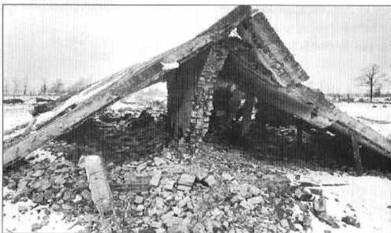
Ruins of Crematorium II, photographed by the Soviets in Feb. 1945, after they had blown it up and blamed it on the Germans. In 2009 it was roped off, with a large sign proclaiming it is undergoing an expensive preservation process.
