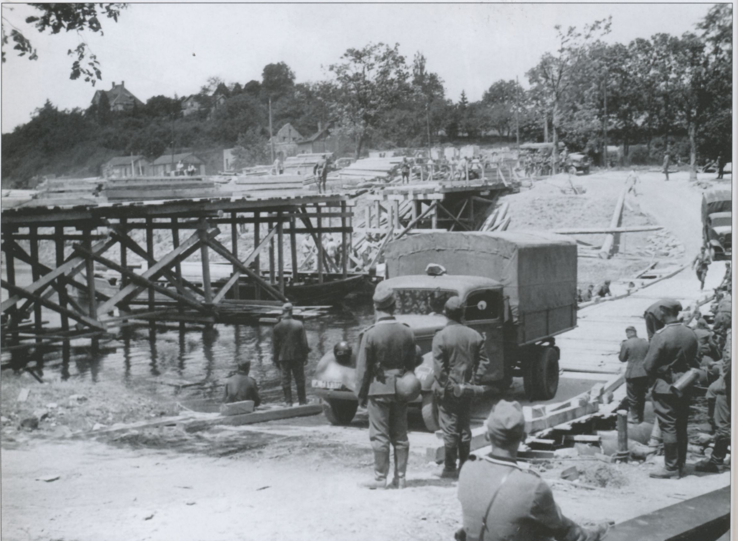
The Germans had to cross numerous water-courses during Barbarossa, none of which seriously slowed them down. The Soviets destroyed many bridges during their retreat. Here a Daimler-Benz L3000 crosses a low-water bridge on the right while construction troops build a new bridge to the left.
