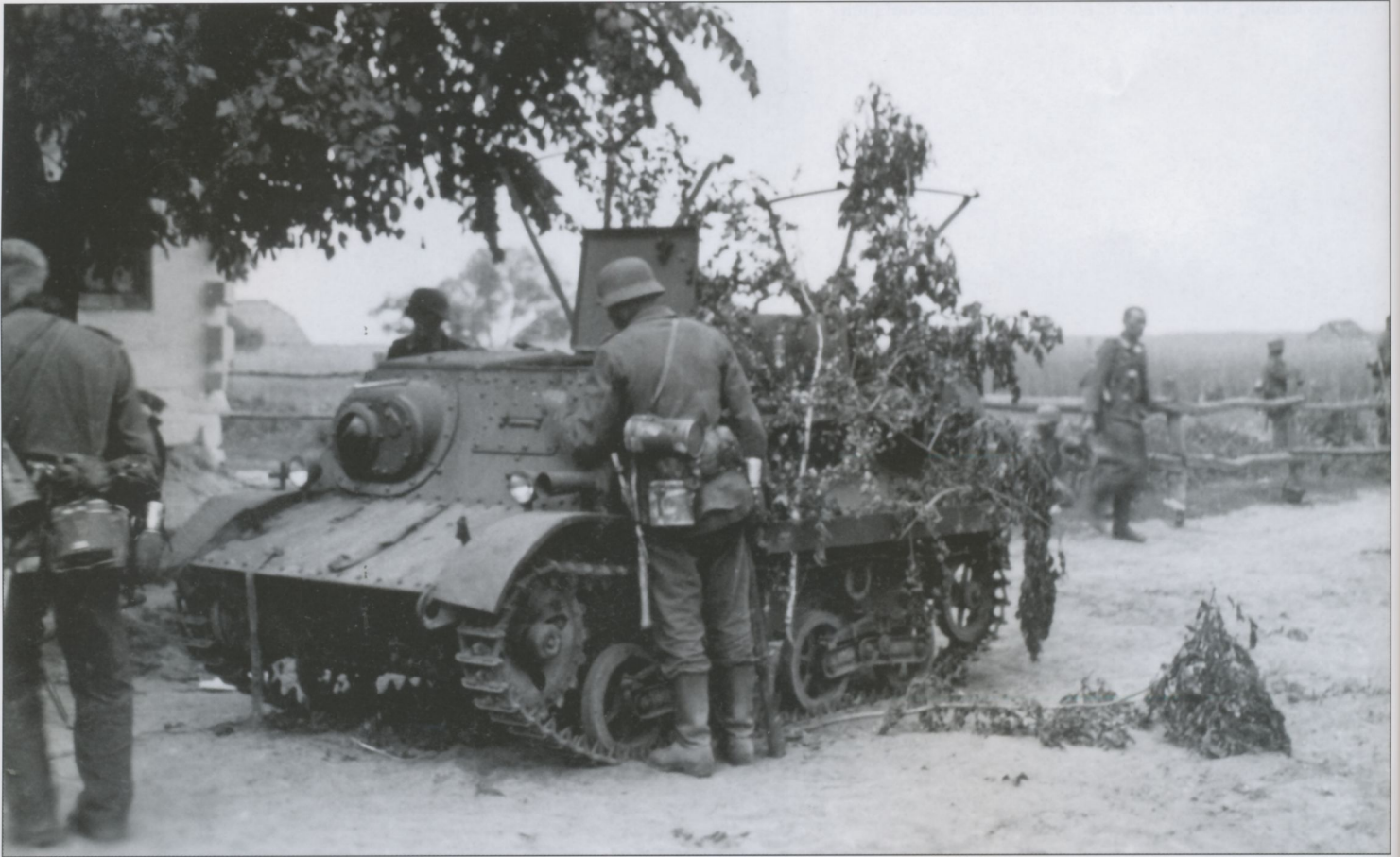
A lightweight STZ-3 Komsomolec artillery prime mover. It had a bow machine gun and seats for the artillery crew.
