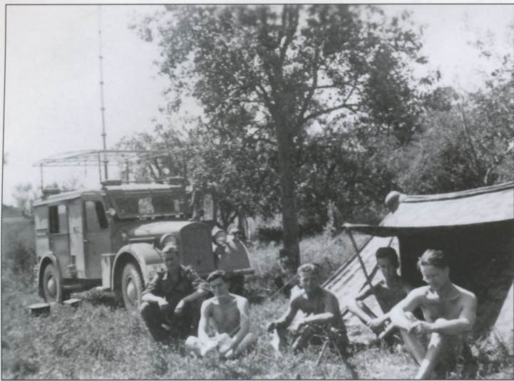
Mobile field communications outpost including truck with built-up compartment and antenna.
