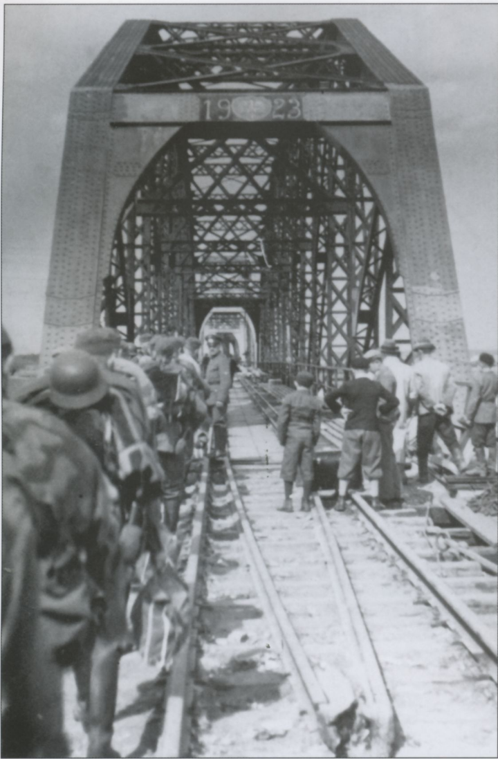
German soldiers march across a railroad bridge while some native men look on. The retreating Red Army failed to destroy many such bridges, which the Germans often captured intact and used to keep their Panzer advancing.
