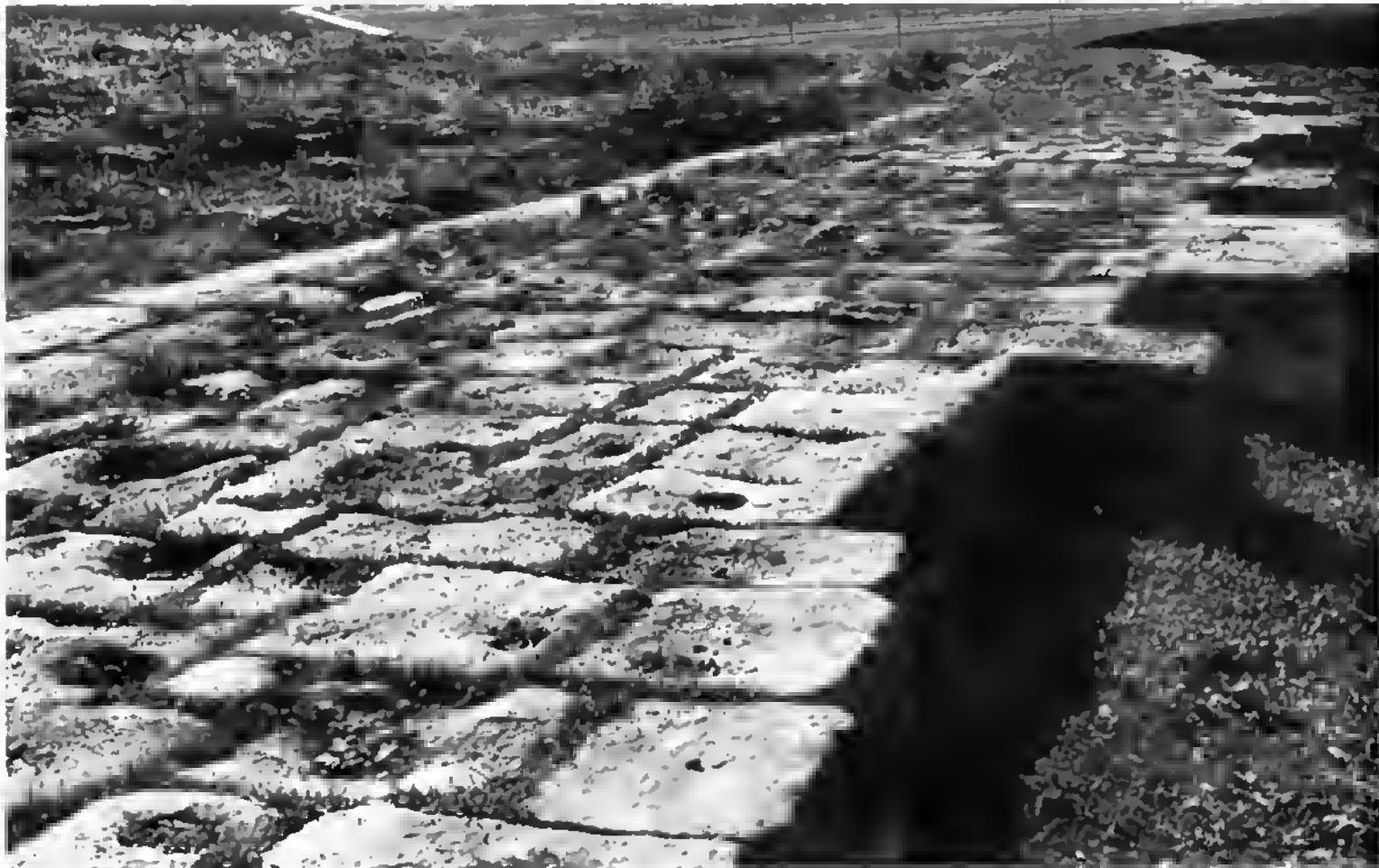
234, 235, 236 The Roman road system was eulogized by contemporaries as the visible sign of the Empire's unity and expansion; a paved road in Syria and, opposite, a milestone a thousand
