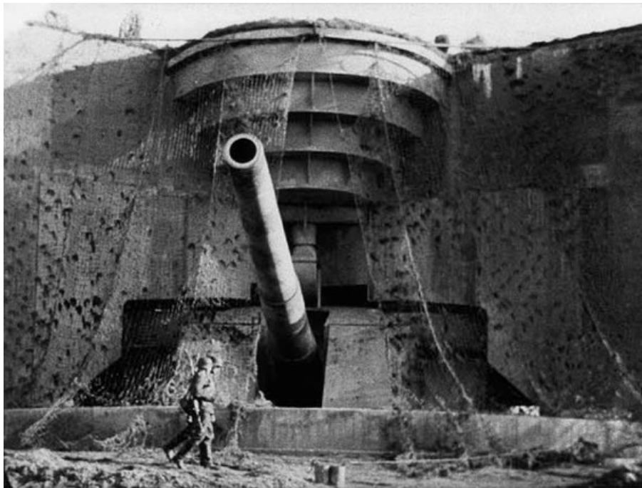
A coastal battery with camouflage netting. During the Normandy invasion, four battleships bombarded a similar gun position at Houlgate. The battery sustained over 1,000 hits, some from 15-inch diameter projectiles and from aerial bombs, without serious damage.
